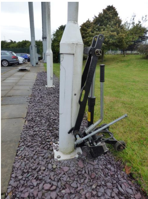
1. Attach counterbalance to column
