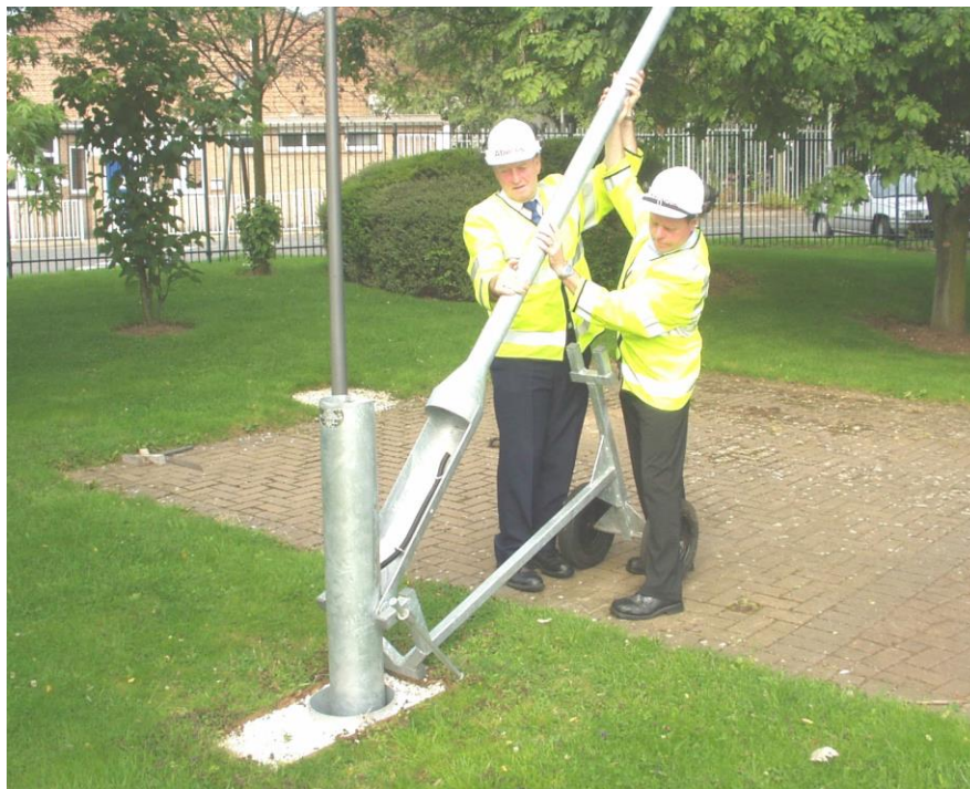
Figure 10-4 - Raising the column to a vertical position
