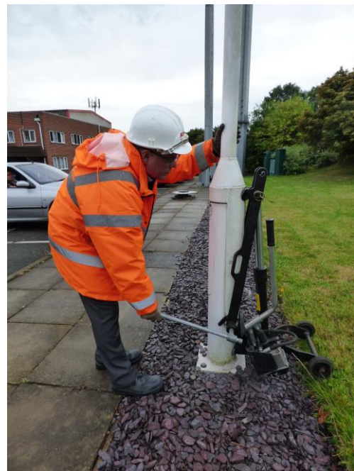
2. Rotate the operating lever
