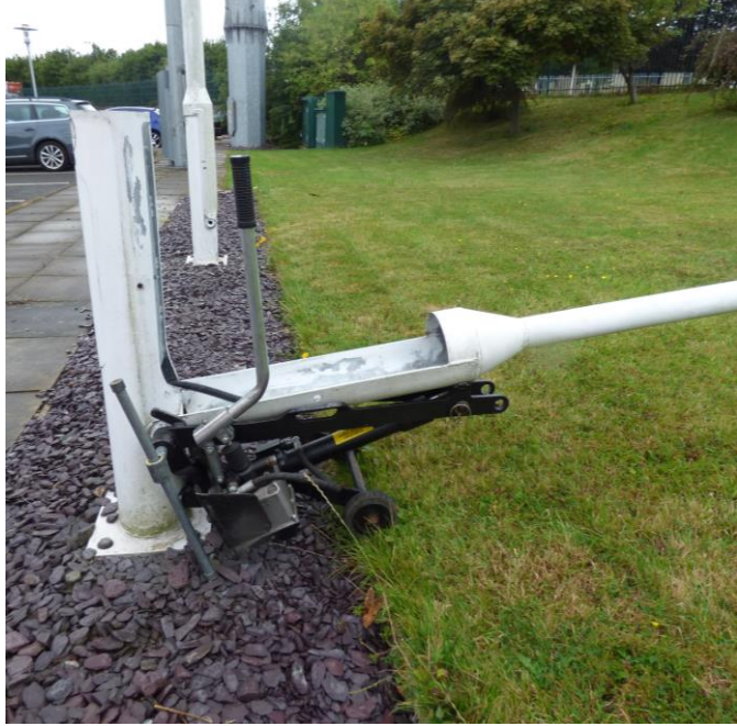
4. Column fully lowered
