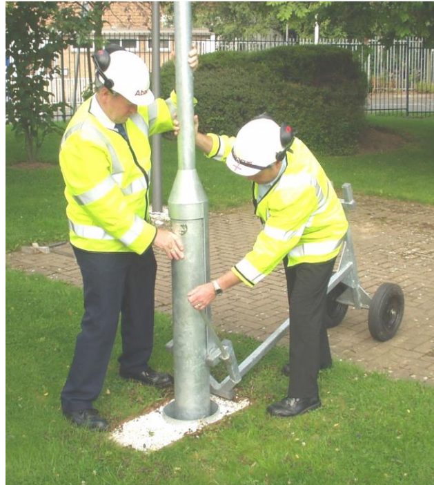
Figure 10-5 - Rotate the operating lever to close the lid
