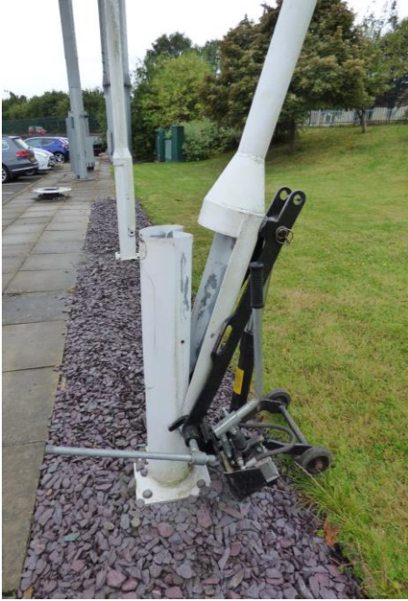
3. Open the control valve to start lowering
