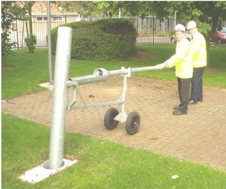
Figure 10-3 - Lowering the root section into the foundation hole
