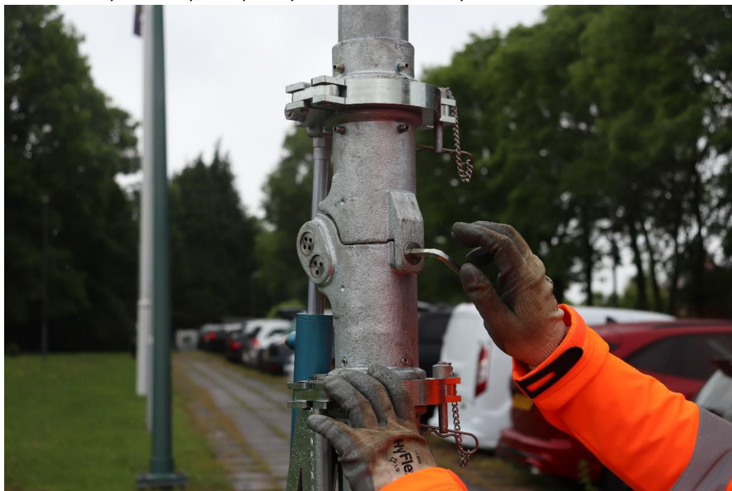
Figure 4 Removing the safety screw
