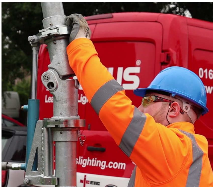
Figure 8 Pushing column in direction of fall
