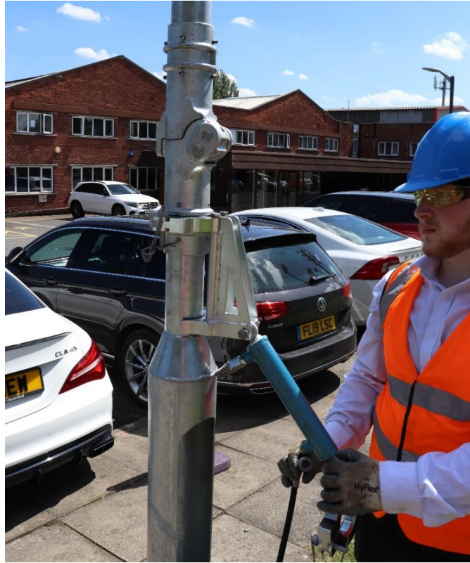
Figure 2 Connecting quick detach hose from pump unit to ram.
