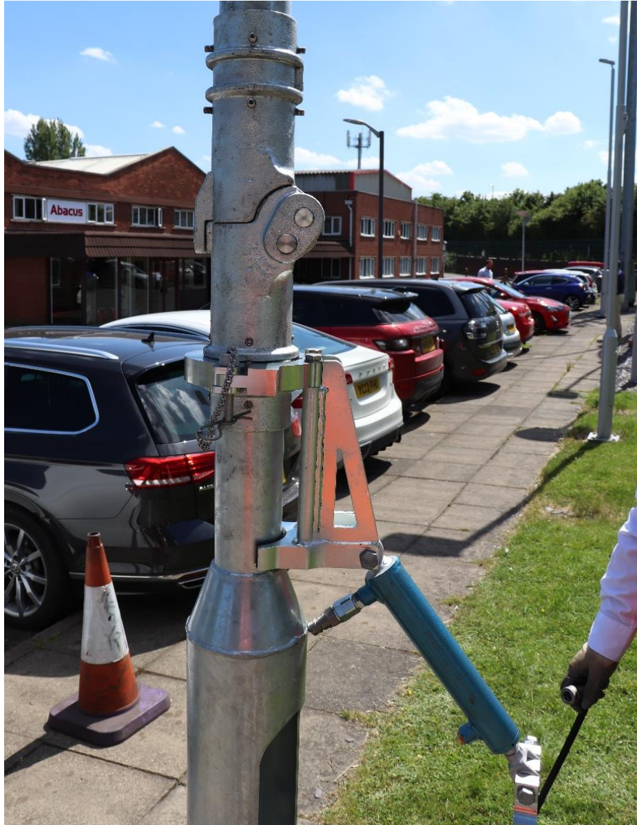
Figure 1 Lower clamp affixed to column. Please note that clamps are keyed to ensure correct orientation
