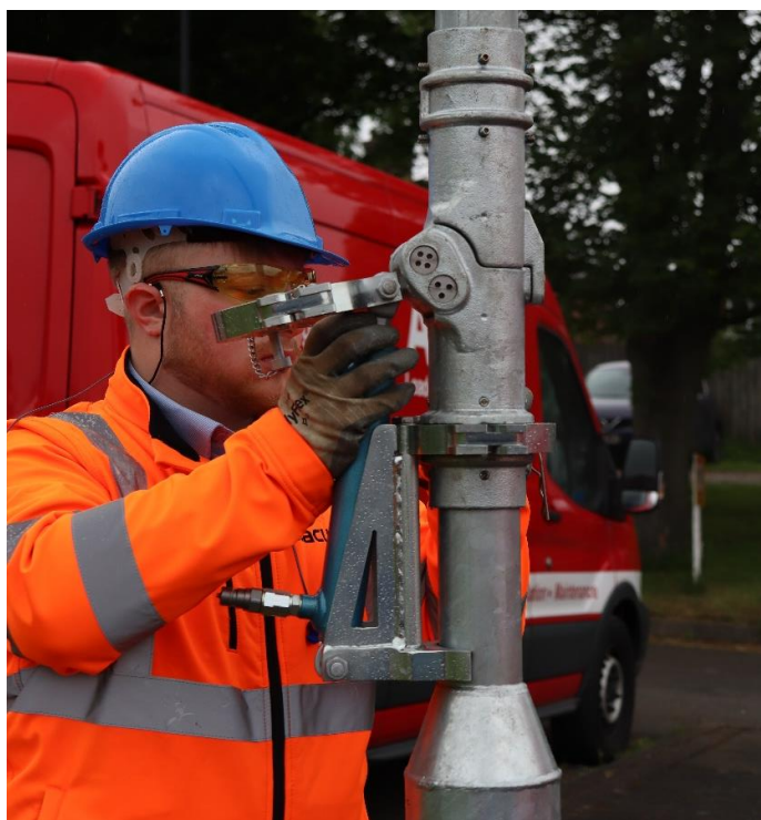
Figure 12 Removing counterbalance
